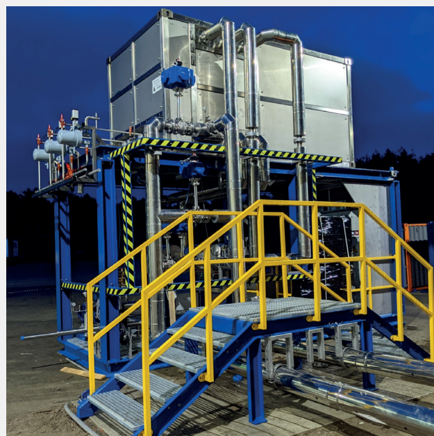
Figure 4: The skid and heat exchanger block connected and installed at Frigologix: (Dohmeyer & Frigologix).
